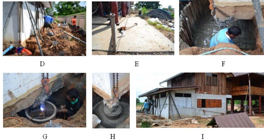
Figure 1 The house lifting process of house no. 1
