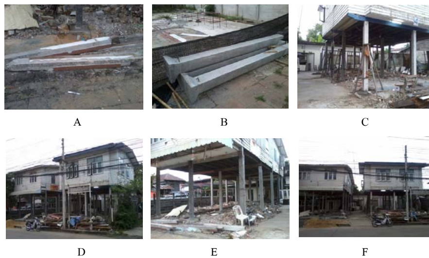
Figure 4 The house lifting process of local technician group no. 4
